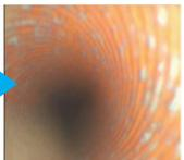
Removing scale adhered to inside of a heat exchanger in a turbo type refrigerating machine (10 months after)
